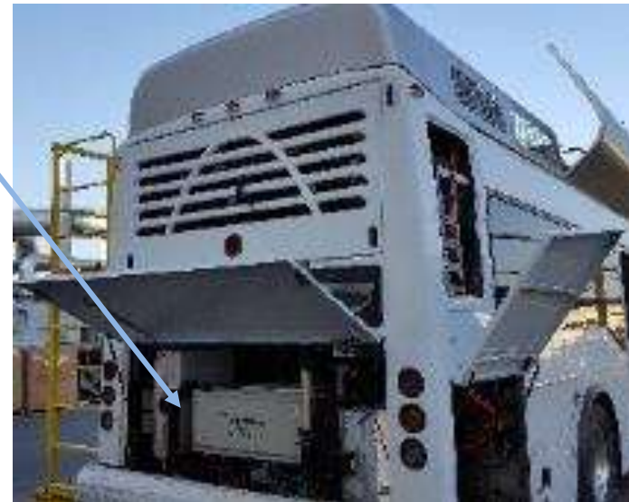
FC engines are installed in the engine bay using OBDII CAN Diagnostic tools
